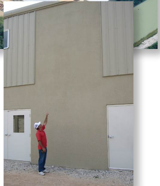
The ArmorCar™ VRC was installed through the roof and then used to move building materials up for final construction of the second level.
